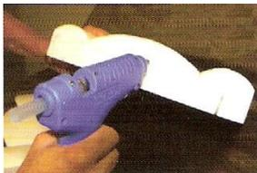
Using the **LOW TEMP GLUE GUN** (do not use a mini or high temp glue gun), apply the glue liberally to the end of one of the extensions that is adjacent to another on your work surface. Line up the front contours of the cornice evenly, and press the two surfaces together for at least 30 seconds. Repeat this process until all of the extensions are glued together.
