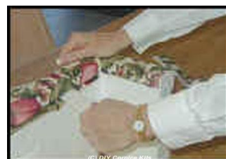
#5- Tuck fabric strip into back tuck groove.
